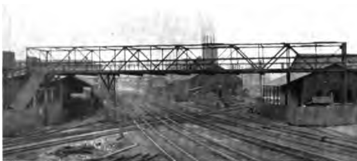
Fig. 2. Viaduct at Plant Entrance.*
